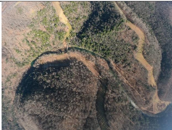
Milepost 74.9 G0024404.jpg Major Stream crossing issues.
