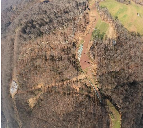
Milepost 47 G0024921.jpg Bare, unvegetated area. Sediment overflowing E&S device near stream crossing. Large slip area that is still unvegetated.
