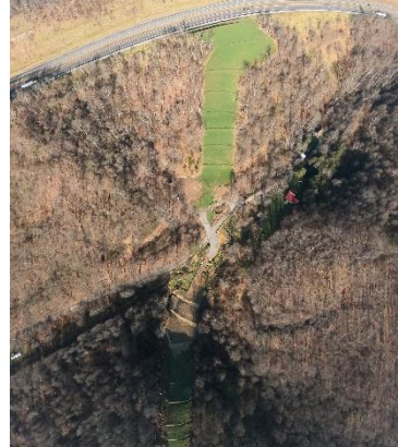
Milepost 60.3 G0024680.jpg Bare dirt next to stream crossing.
