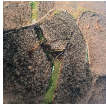
Milepost 55.2 G0024770.jpg Problem area south of Copley Rd. ROW and triangular workspace area in shadow show collapsing slopes and sediment in stream crossing.
