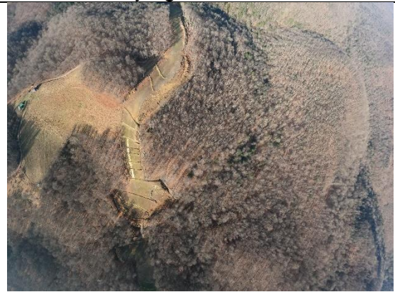
Milepost 77.9 G0024350.jpg Bare areas by top water bars, piles of dirt/sediment
