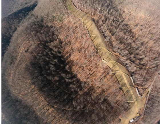
Milepost 80.2 G0024312.jpg Possible washouts through woods, sediment piles
