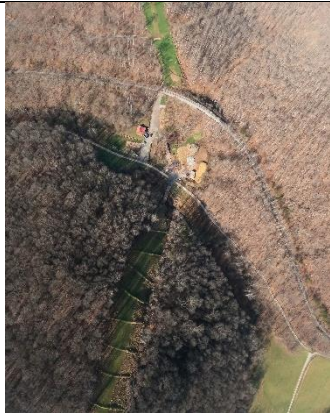
Milepost 65.5 G0024584.jpg Construction area. Bare unvegetated areas next to stream.
