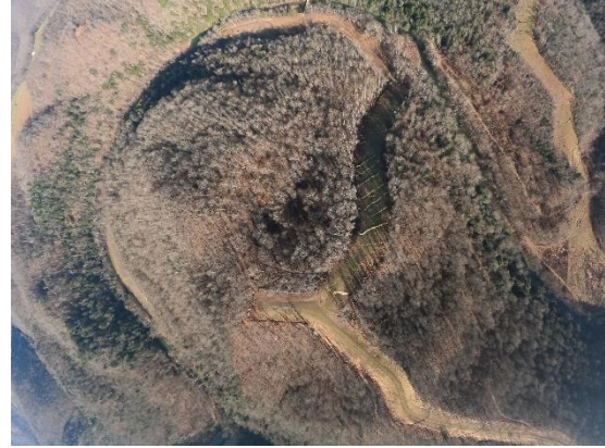
Milepost 75.1 G0024401.jpg Bare areas next to stream crossing. Erosion devices appear to be missing.
