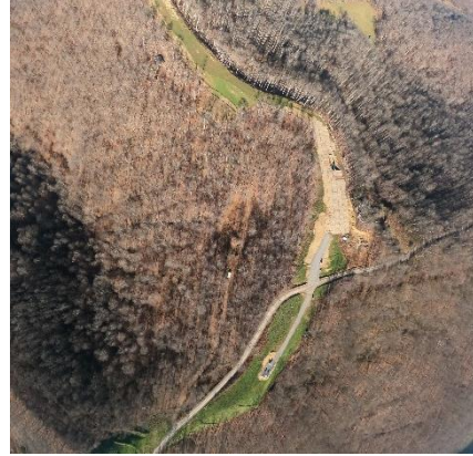
Milepost 52.8 G0024810.jpg Large timber mat surface with slip and erosion control measure failure
