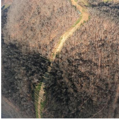
Milepost 59.4 G0024695.jpg Large bare, unvegetated areas, E&S measures need maintenance.
