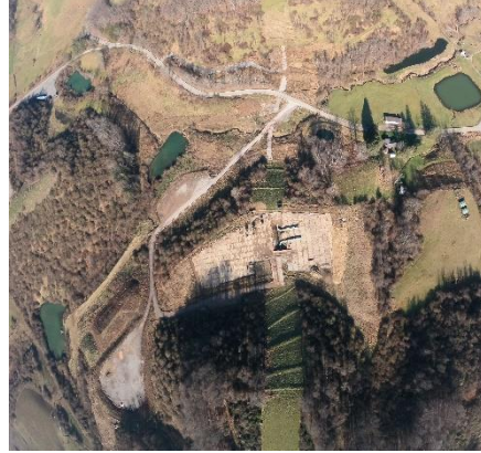
Milepost 45.9 G0024942.jpg Large timber-matted work area south of Churchville Rd/CR-9 crossing. Sediment in stream below road crossing.
