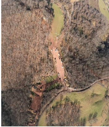
Milepost 46.5 G0024931.jpg Unvegetated areas with sediment flowing off LOD.
