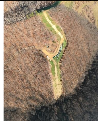
Milepost 43.0 G0024996.jpg Unvegetated area at bottom slope is eroding into stream.
