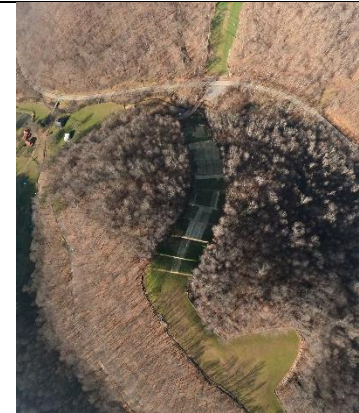
Milepost 62.2 G0024643.jpg Extensive matting shown with slips at MP 62.3 on 10/15/20, 10/29/20 and 12/5/20.
