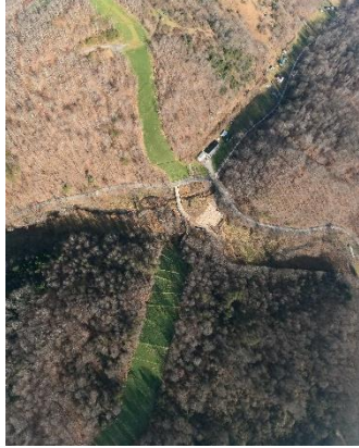
Milepost 68.7 G0024524.jpg Muddy construction area/water crossing, timber mats
