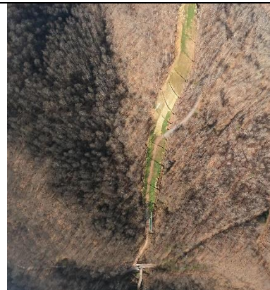
Milepost 61.1 G0024664.jpg Large area of bare soil on slopes with matting.
