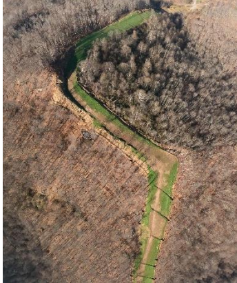
Milepost 60.6 G0024673.jpg Unvegetated areas with signs of slip on slope.
