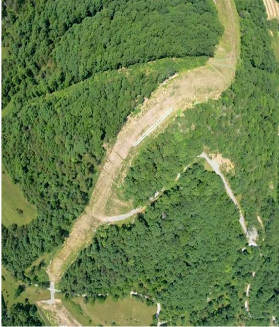
Milepost 185.3 Exposed soil on slope.
