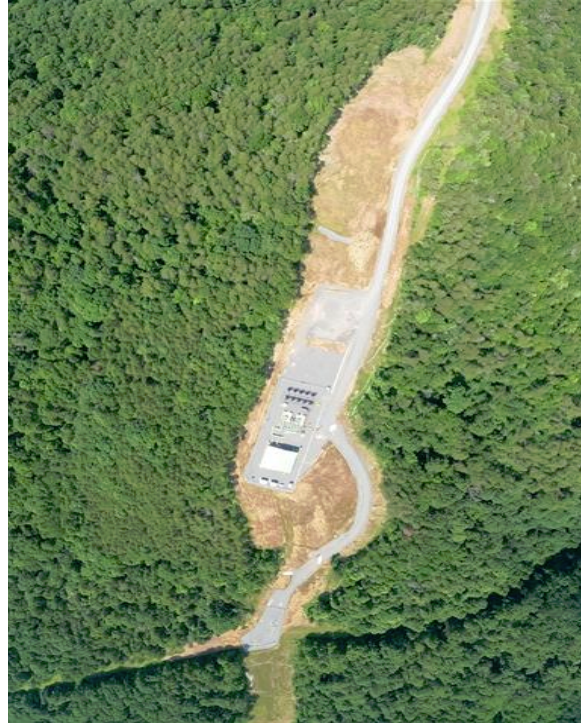
Milepost 180.7 Large area needs additional seeding.
