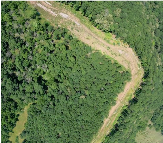
Milepost 189.7 Additional seeding needed on exposed areas.
