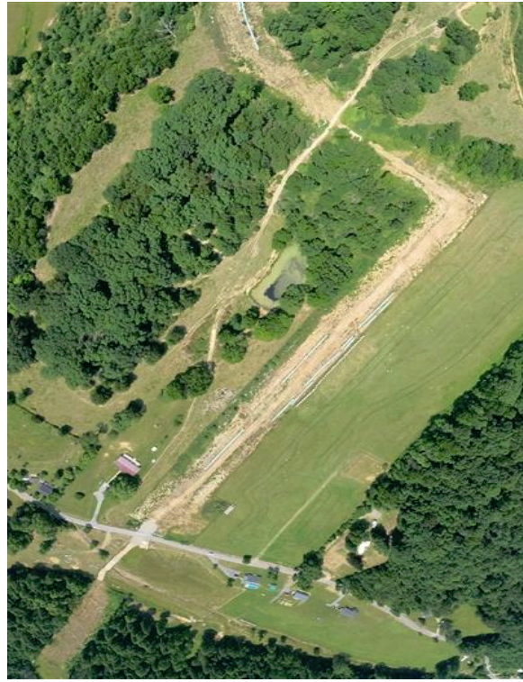
Mileposts 191.8 - 192.1 Large area of exposed soil in ROW. Additional seeding needed.
