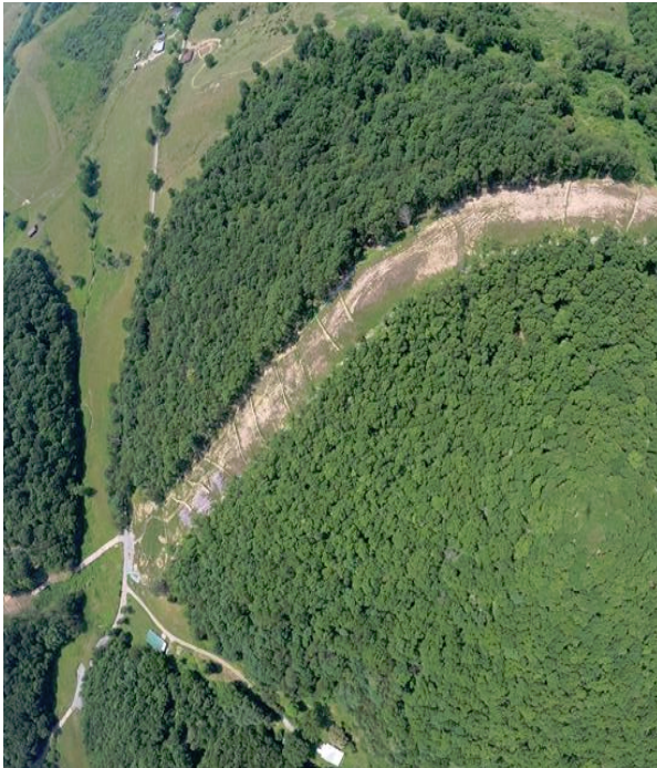
Milepost 194.3 - 194.6 Numerous bare areas on slope above Painters Creek.
