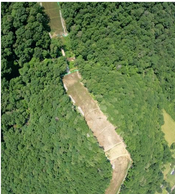
Milepost 187.7 Exposed soil on slope on other side of Narrows of Hans creek crossing.
