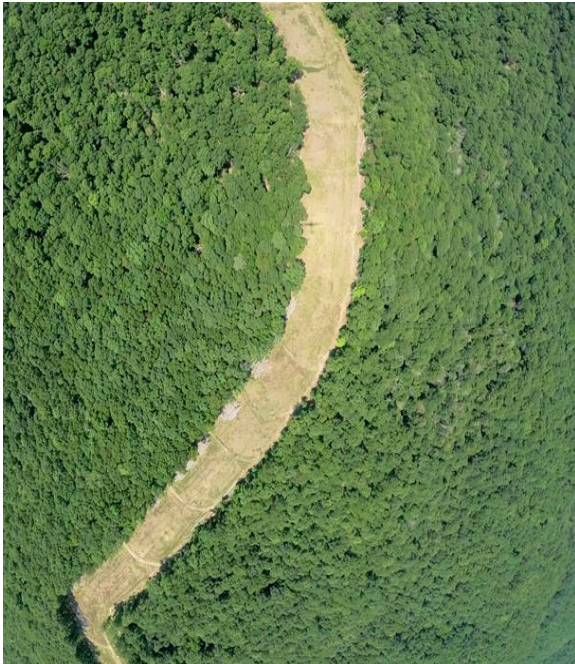
Milepost 181.7 Exposed soil on ridgeline.
