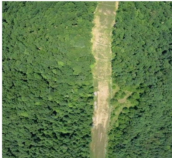
Milepost 178.8 Exposed soil needs additional seeding.
