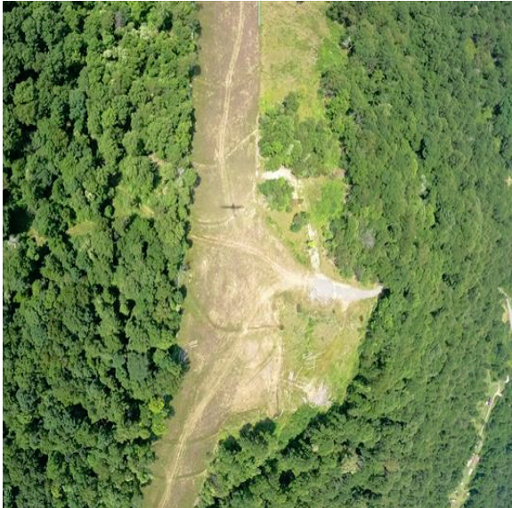
Milepost 187.4 Exposed soil at ATWS needs additional seeding.
