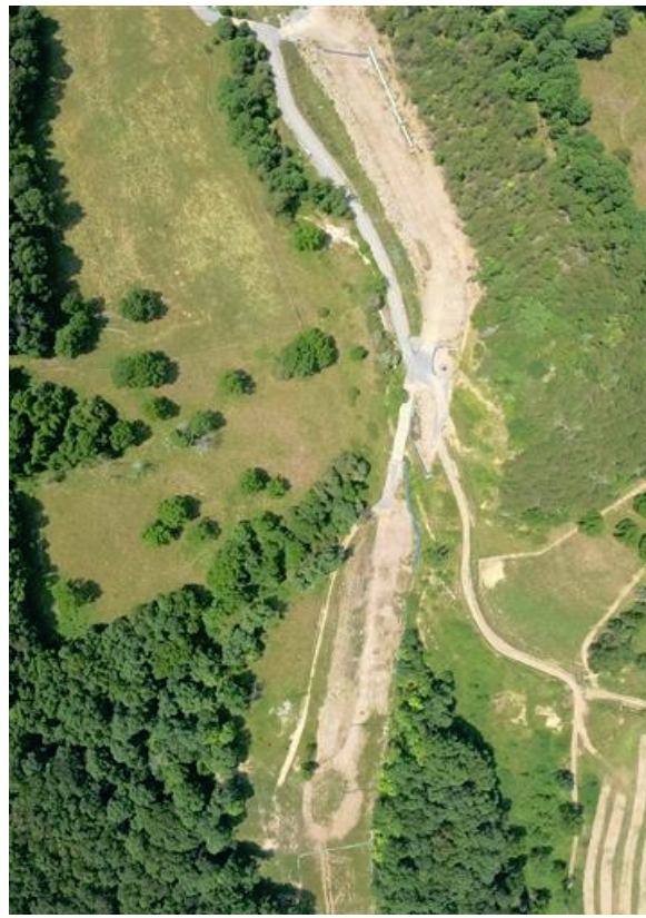
Mileposts 184.2 - 184.4 Exposed soil next to creek lacks vegetative cover.
