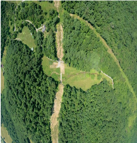
Milepost 172.7 Exposed soil next to Kellys Creek and Kellers Creek road.
