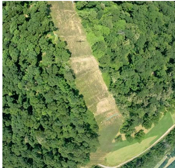
Milepost 186.3 Bare spots on slope
