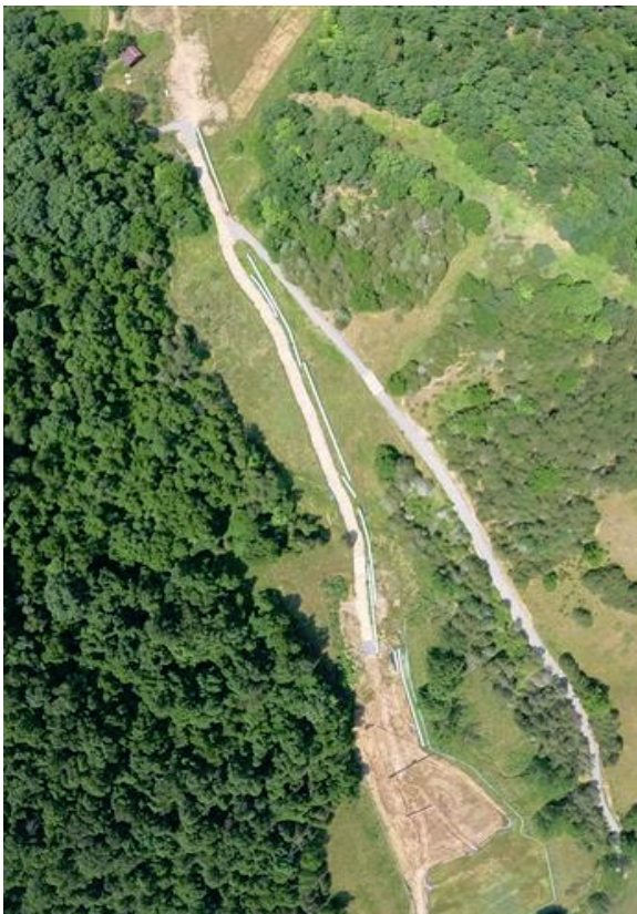
Mileposts 182.4 - 182.8 Two large areas of bare soils next to Slate Run.
