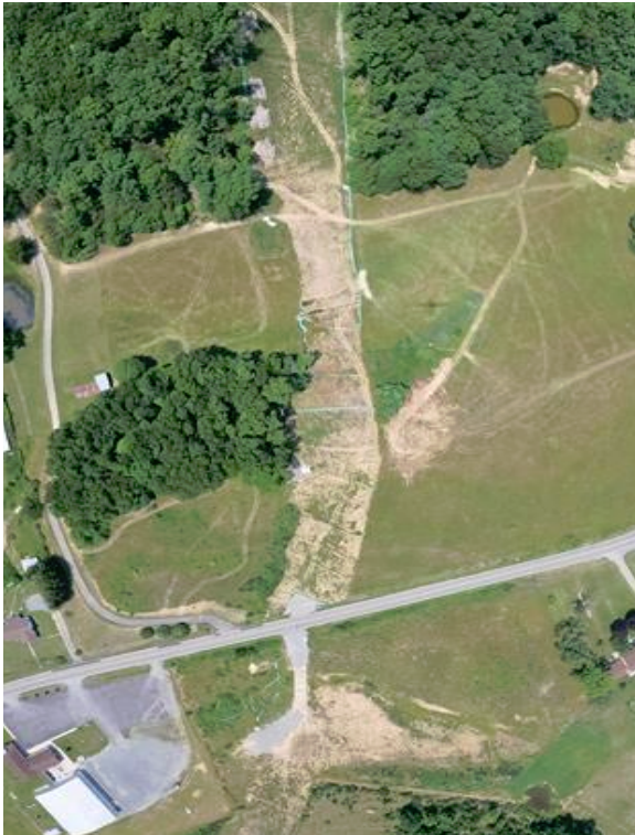
Milepost 191.5 Bare, exposed soil on both sides of Seneca Trail. Reseeding required.
