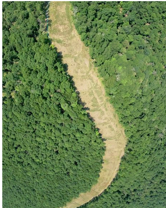
Milepost 181.6 Inspect area to determine if vegetation coverage is adequate.
