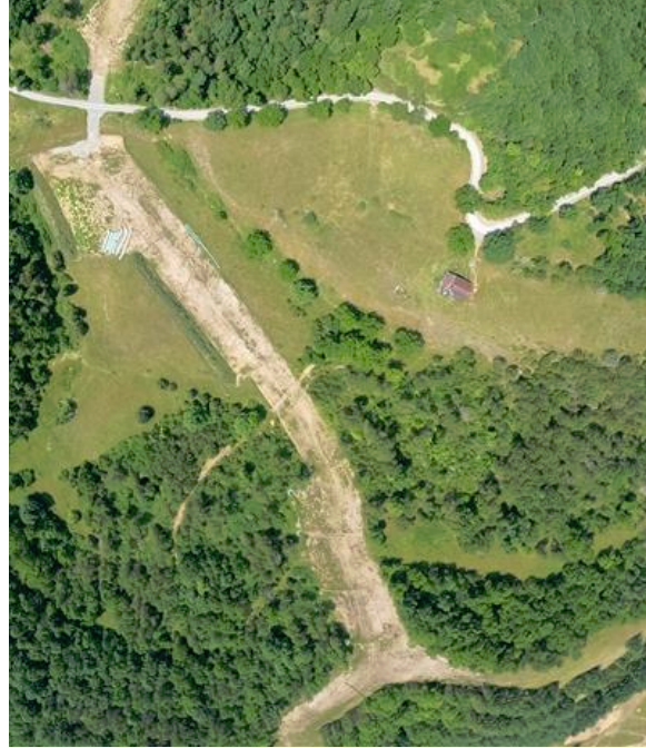
Milepost 185.5 Area with bare soils needs additional seeding.
