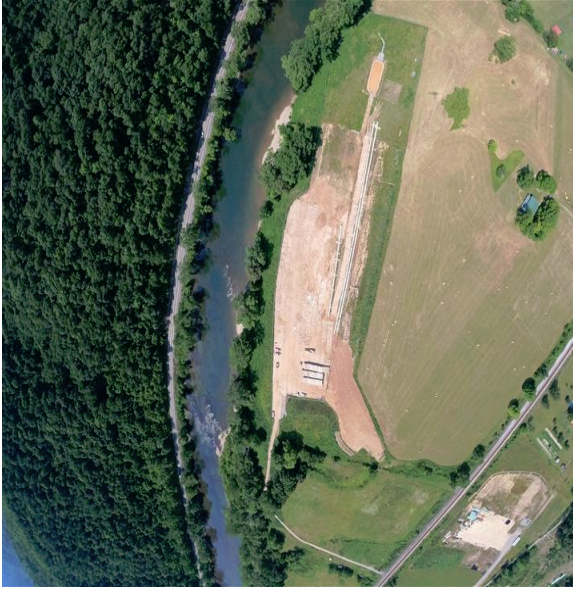
Milepost 171.7 Large denuded area adjacent to Greenbrier River. Sediment deposits are visible on the edge of Greenbrier River.
