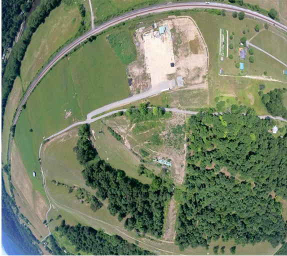
Milepost 172 Laydown yard has lain dormant for over a year with exposed soil.
