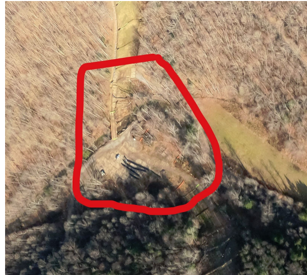
Milepost 82.3 G0024276.jpg Perimeter controls for large bare area are at the edge of stream crossing, instead of setback from stream bank. This area needs stabilization measures installed. Inspection requested.
