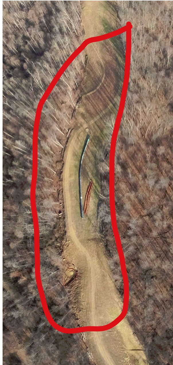
Milepost 89.2 G0024162.jpg Bare unvegetated areas on the ridge line. Seeding maintenance needed at this location.
