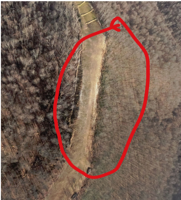
Milepost 94.6 G0024071.jpg Remote location at the top of the ridge has sparse vegetation. Perimeter erosion controls are not visible. Inspection requested.
