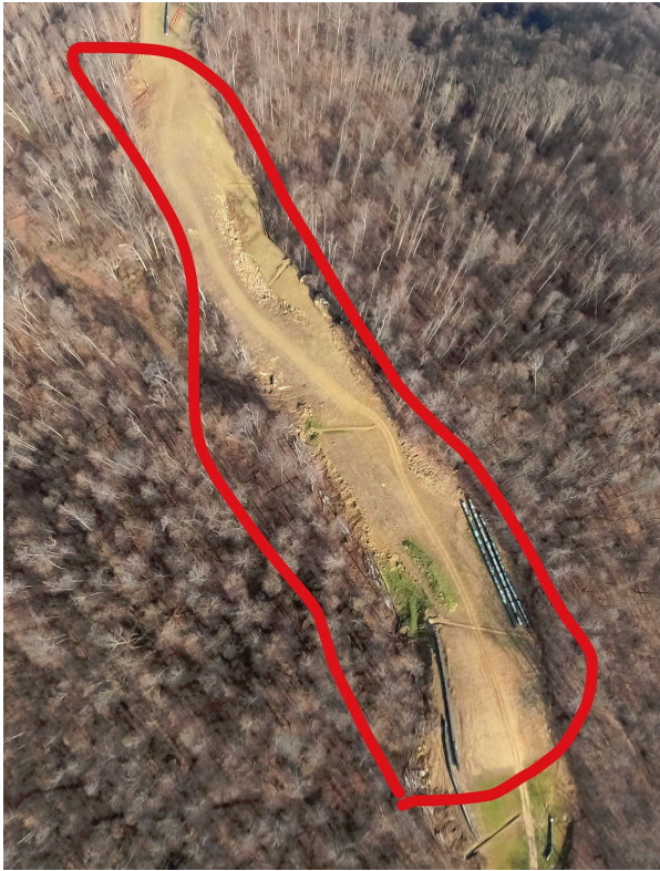
Milepost 89.4 G0024159.jpg Large unvegetated area on the ridge line. Inspection and seeding requested.
