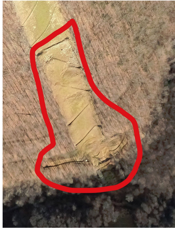
Milepost 92.4 G0024109.jpg Large unvegetated areas adjacent to stream crossing on both sides. Rill erosion occurring on the slope above the stream. Possible slips forming on slope at this location. Inspection requested.
