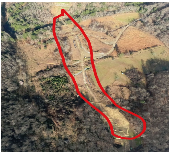
Milepost 81.8 G0024285.jpg Several areas without vegetation cover next to stream crossings.
