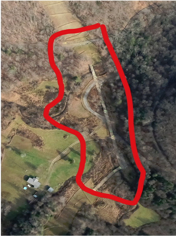
Milepost 93.1 G0024095.jpg Stream crossings. The area at the bottom of slopes is not well protected. Erosion control devices are not visible. Too many unvegetated areas close to the stream. Pipeline has no stream buffer at the stream crossings.
