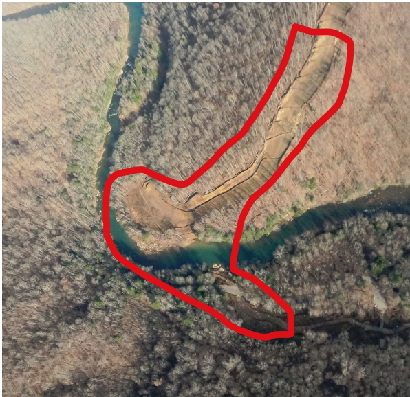
Milepost 87.2 - 87.4 G0024192.jpg Large area with no vegetative cover next to river crossing. There is evidence of sediment flowing out of ROW, This area needs inspection.
