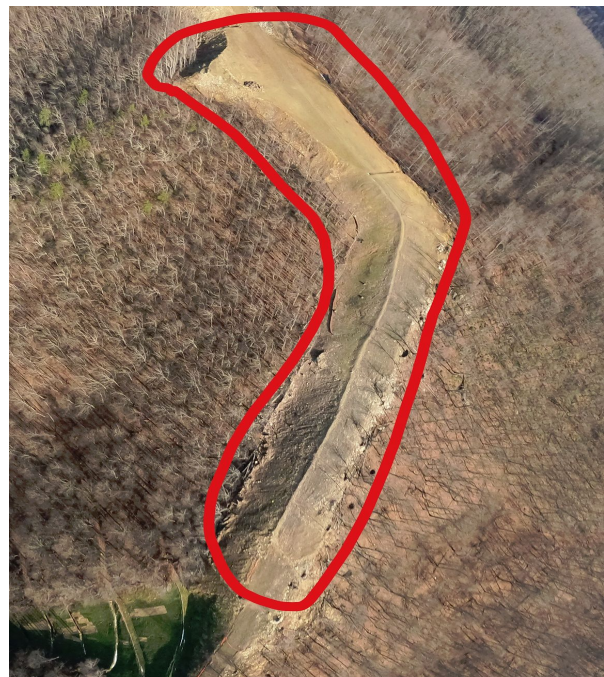
Milepost 86.7 - 86.6 G0024205.jpg Large area with little vegetation on top of ridge. Remote location that needs inspection. It looks like the erosion control devices require maintenance.
