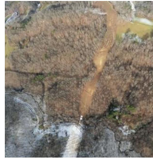
Milepost 149.8 G0023098.jpg Bare/sparsely vegetated areas with rill erosion creating possible slips. Re-seeding required to stabilize slopes.
