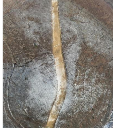
Milepost 142.2 G0023234.jpg Long slope with bare/sparsely vegetated areas. Re-seeding required to stabilize slope.
