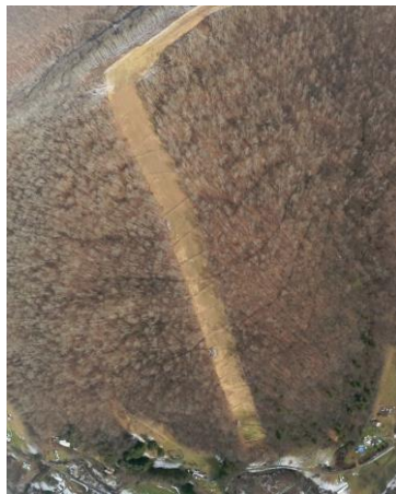
Milepost 146.6 - 146.9 G0023156.jpg Long steep slope with bare/sparsely vegetated areas and rill erosion. Re-seeding required to stabilize slopes.
