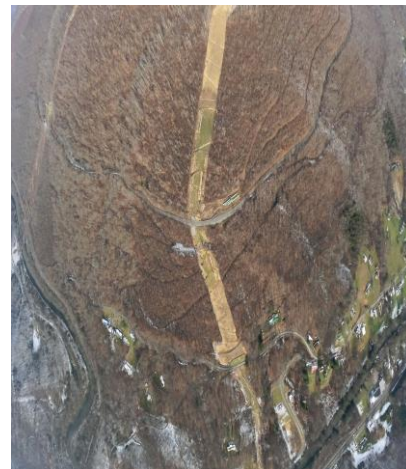
Milepost 143.5 - 143.8 G0023210.jpg Long steep slope with bare/sparsely vegetated areas and rill erosion. Re-seeding and erosion control matting required to stabilize slopes.
