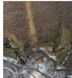
Milepost 147.0 - 147.1 G0023152.jpg Bare/sparsely vegetated areas with rill erosion at toe of slope. Re-seeding required to stabilize slopes.
