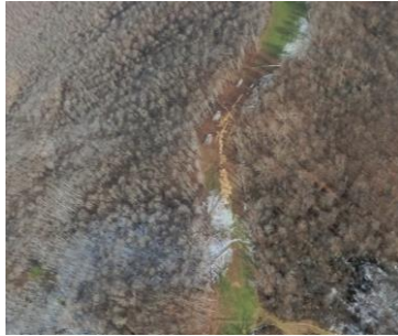
Milepost 150.9 G0023076.jpg Bare/sparsely vegetated area at bend of ROW. Re-seeding required.
