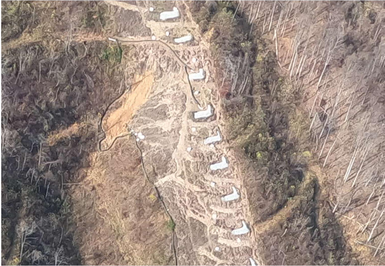
Large slip area shown in photo near milepost 250.8.
