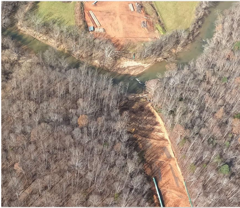
Milepost 269.8 shows a large graded area with little vegetation on both sides of the Blackwater River crossing.
