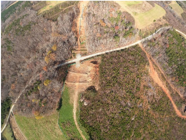
Milepost 286.6 shows bare areas and areas with vegetated cover. There is a stark contrast between the two areas.
