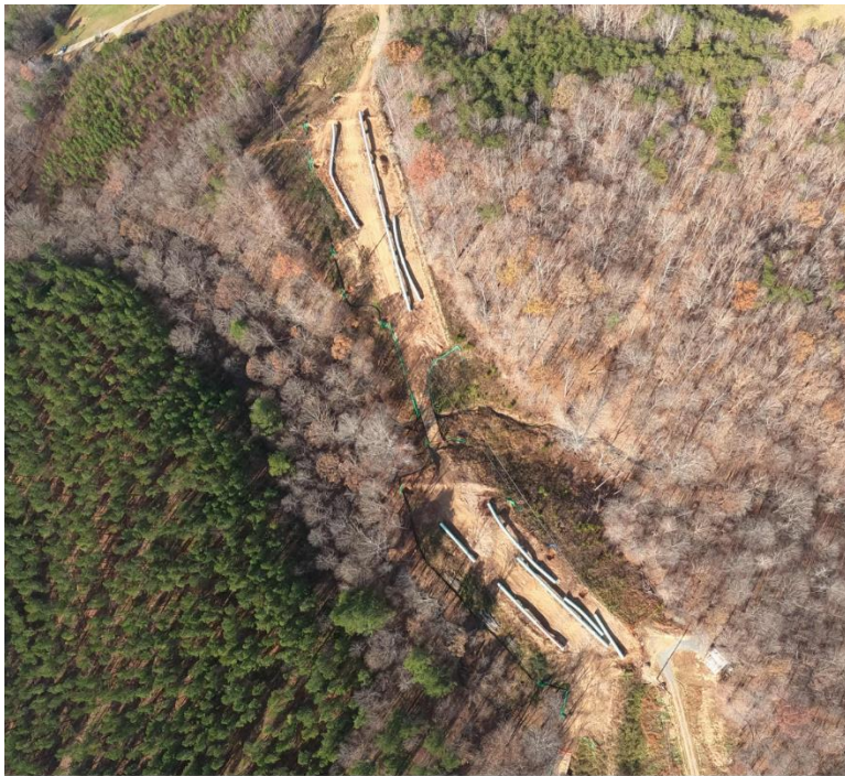
Milepost 279.9 shows bare areas adjacent to Little Jacks Creek.
