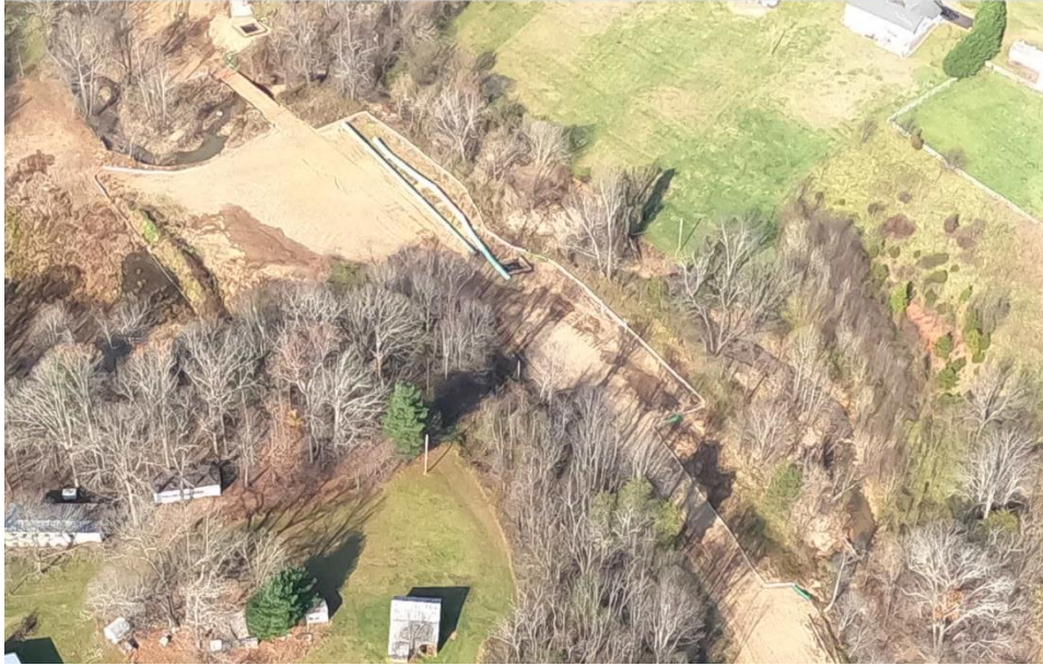
Another shot of Milepost 260.3 at Teels Creek. The LOD of the cleared area is too close to stream. Photo shows LOD at top of bank of Teels Creek.
