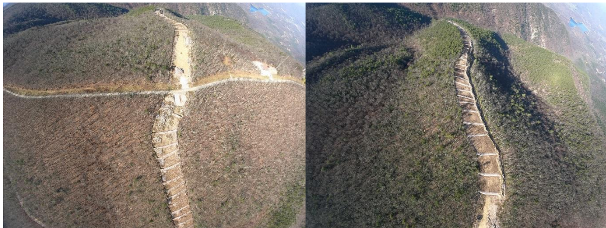
November 21 flight photos at top of Poor Mountain in Roanoke County shows little vegetative cover. Jute mesh blankets were placed months ago, but show little sign of grass growing.
