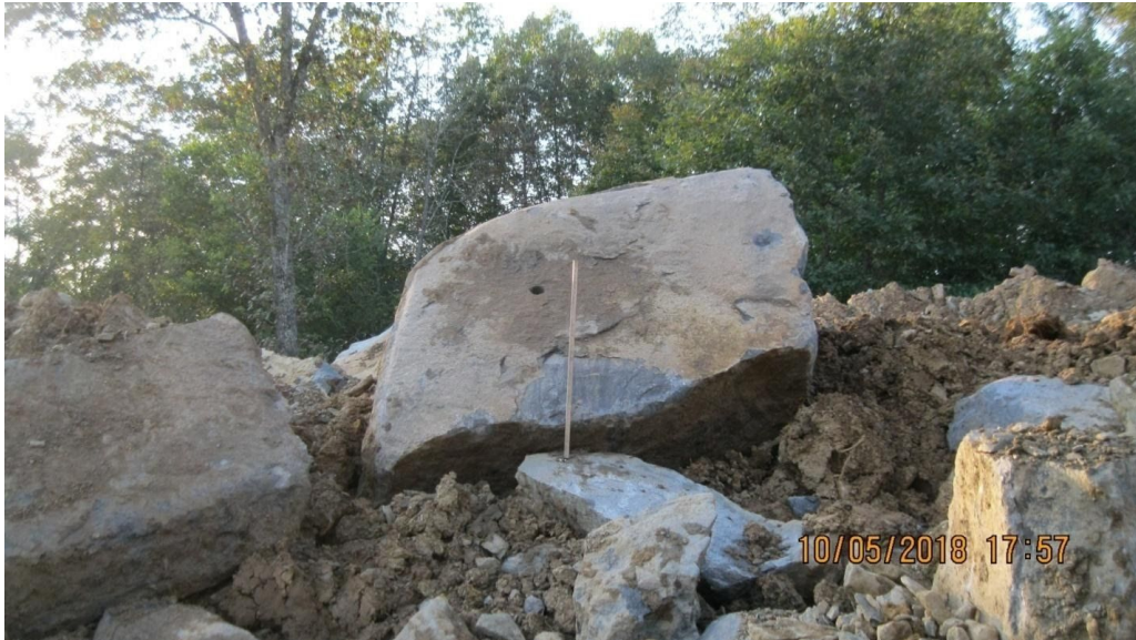
Figure 17: Large carbonate boulder blasted from trench.
