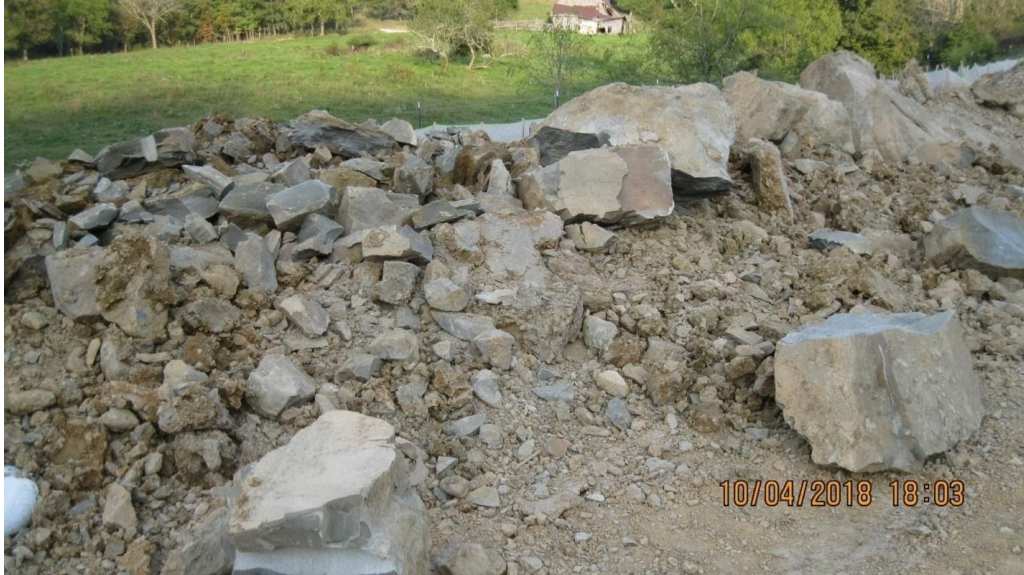
Figure 19: Limestone boulders and rock strewn along right-of-way.
