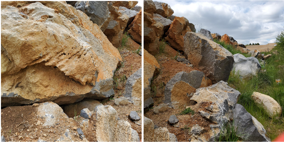
Figure 1B: Blasted limestone strewn along MVP ROW.
