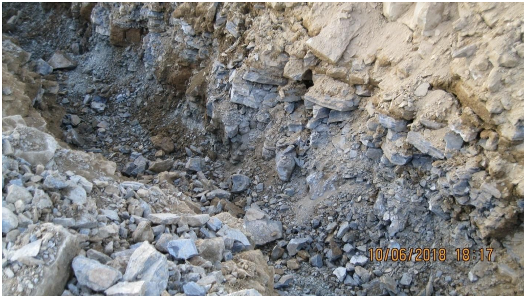
Figure 20: Layers of limestone shown in blasted trench.
