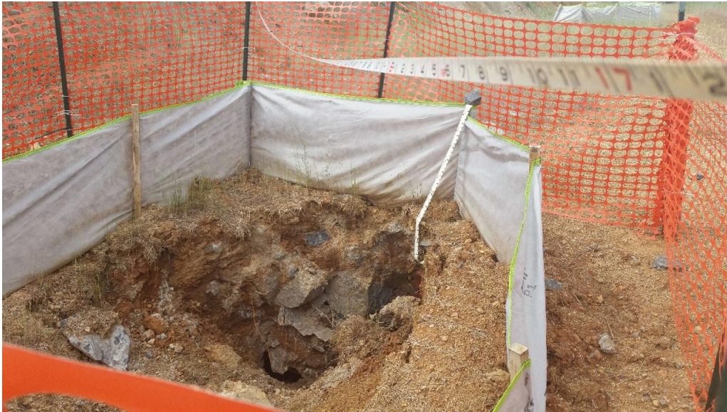
Figure 7: June 2019 site visit shows expanding subsidence in the same location shown in Figure 5.
