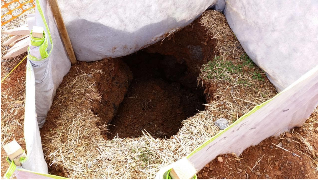
Figure 13: Photo of sinkhole enclosed by silt fence and safety fence.
