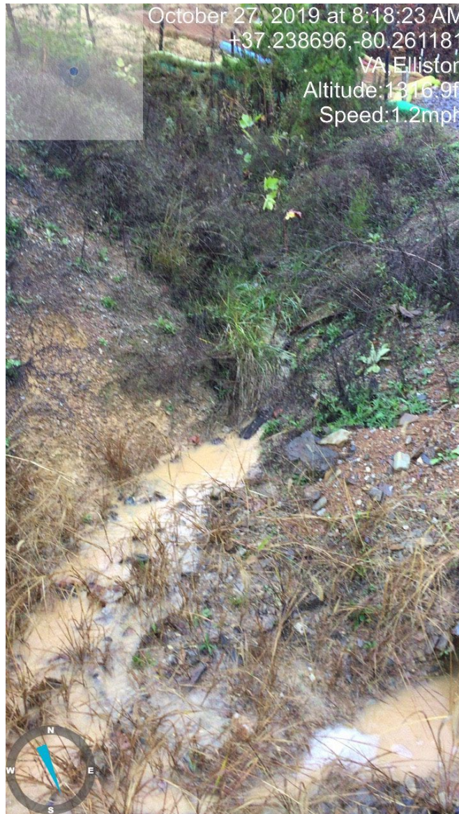
Figure 4: Sediment laden runoff flowing from MVP Right of Way.
