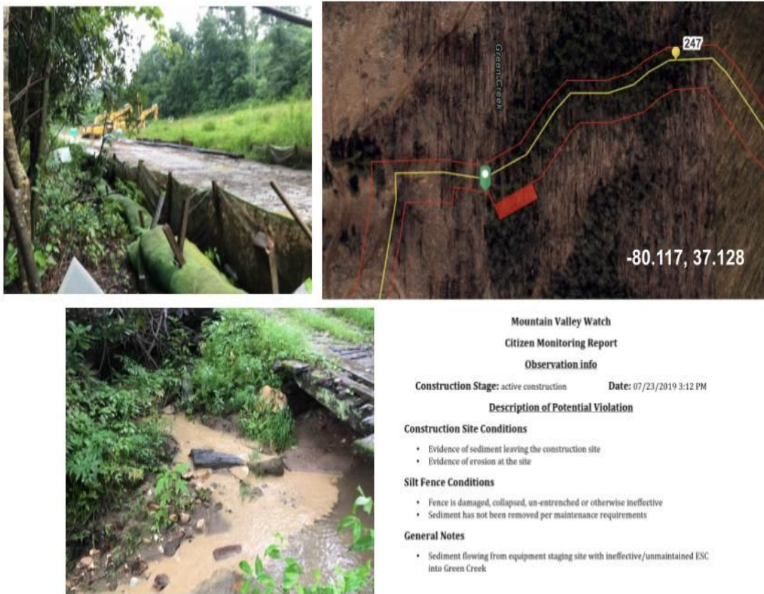
Figure 9. Images of sedimentation to Green Creek July 23, 2019, with an excerpt from the report submitted to DEQ.
