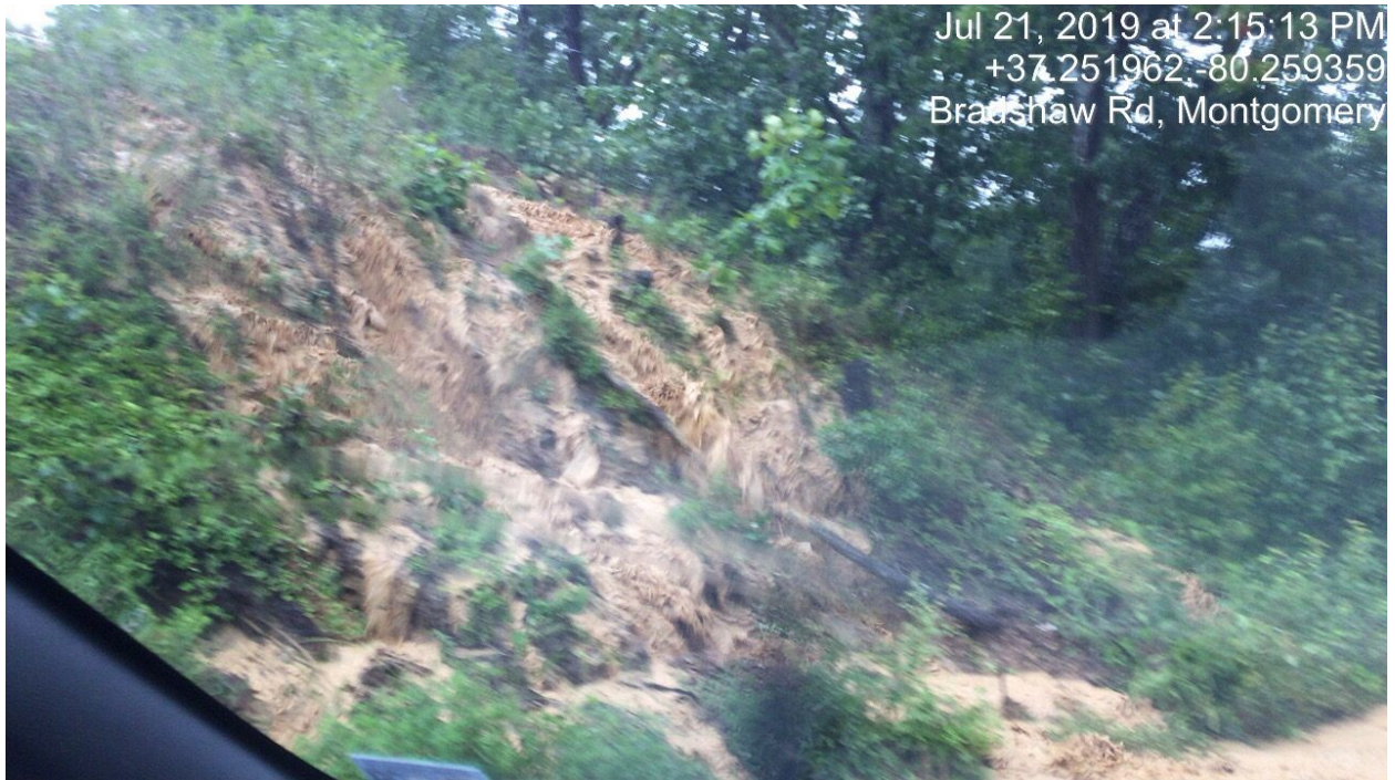
Figure 3. Runoff gouging gullies in steep slopes.
