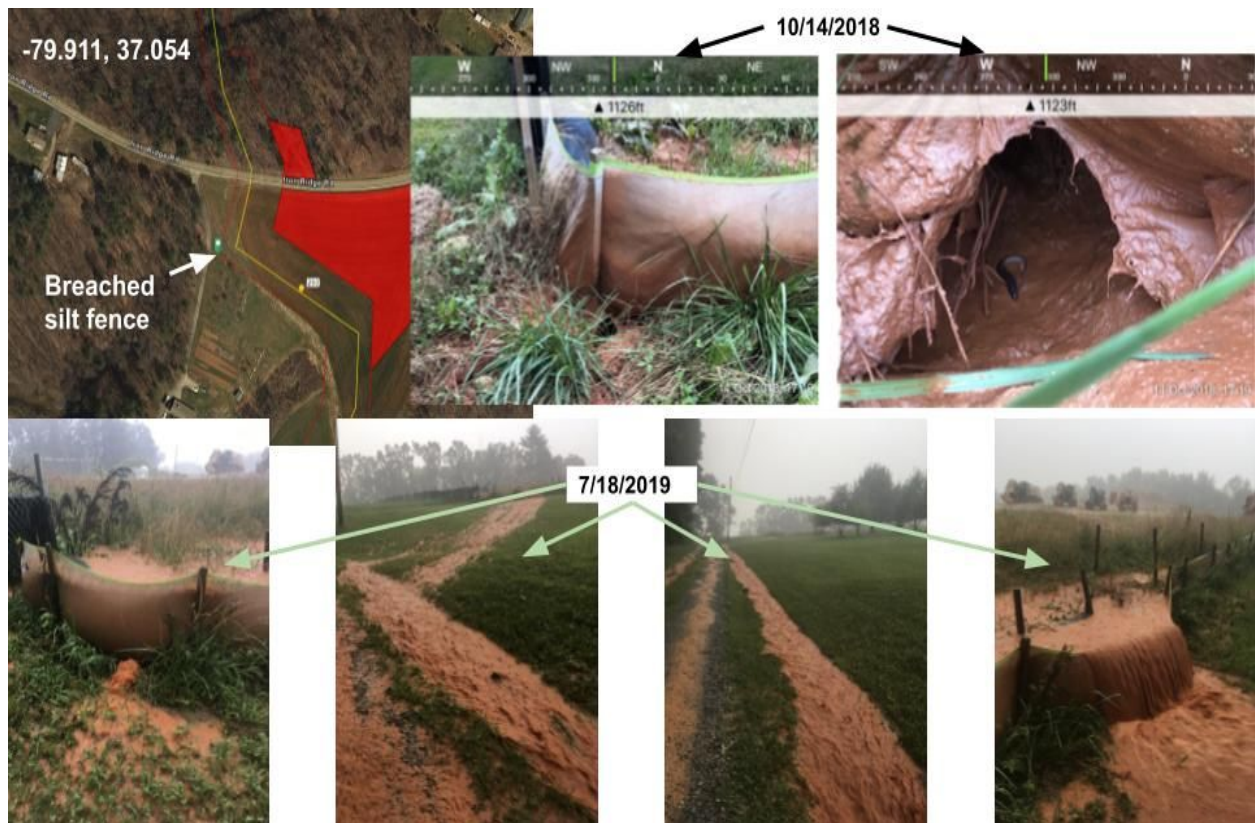
Figure 10. History of sedimentation at the Angle Farm, with images from October 2018 and recent sedimentation event of July 2019.
