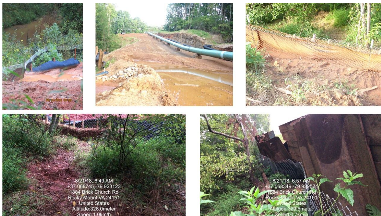
Figure 5: Ground support images. Pallets and plywood sheeting used as sediment barriers.
