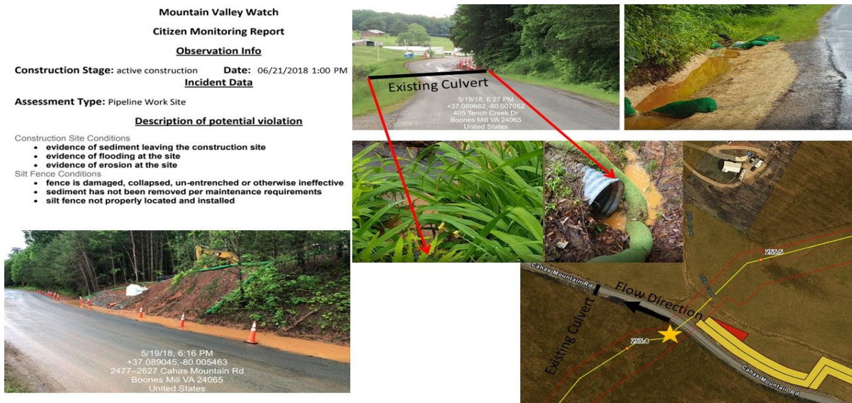
Figure 9: Cahas Mountain Road mudslide site showing location of sediment entry to Little Creek through an existing culvert beneath road.
