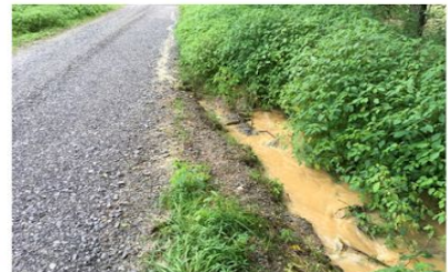
This is 05 Aug at 15:08 hr . Sediment is still still entering stream at damaged bank.
