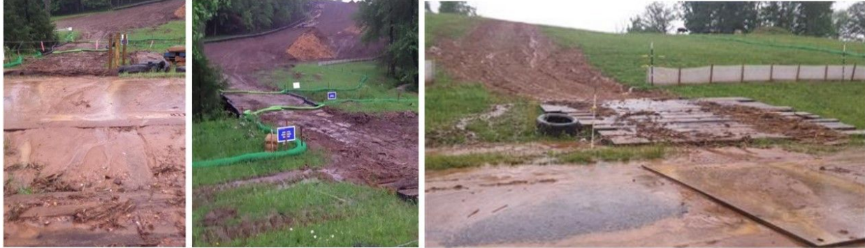
Figure 16: Potential violations reported May 18, 2018
