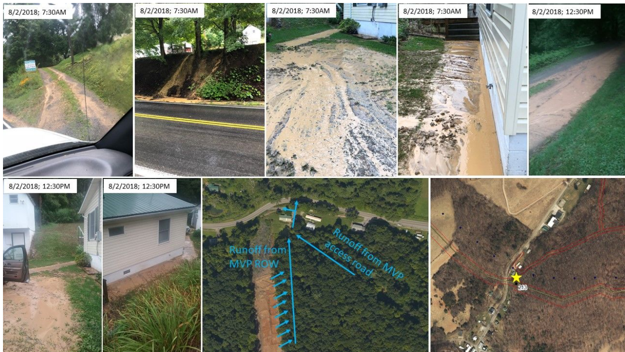
Figure 32: Photos from August 2, 2018 reported incident in Historic Newport.
