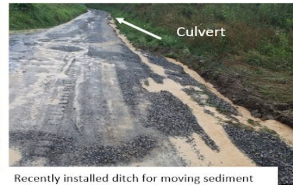
Recently installed ditch for moving sediment off worksite. Unfortunately, ditch is (purposefully) connected to a culvert intended to drain water from grassed bank (with no erosion). Now sediment entering culvert moves directly, with no BMPs in place, into the stream. Culvert is at the far end of this photo
