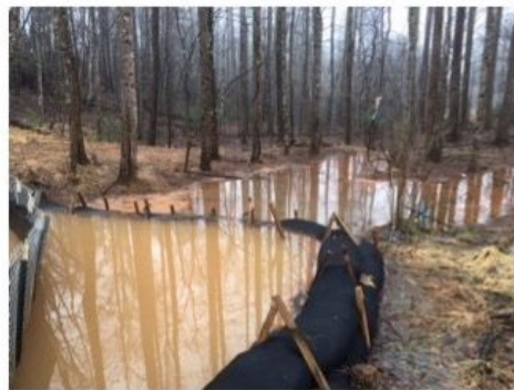
Figure 5: Images showing muddy water overrunning silt socks at the Cahas Mountain Road crossing in late February 2019.
