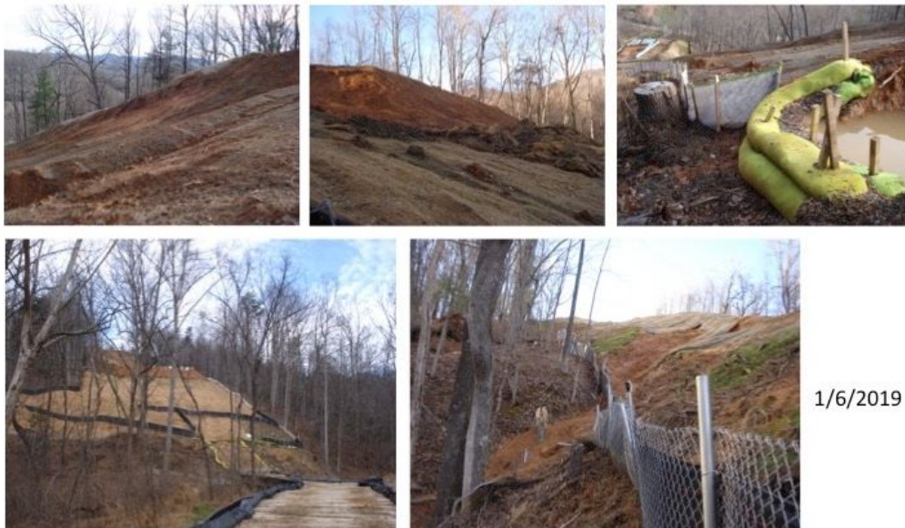
Figure 4: Lack of adequate slope stabilization and ESC maintenance was reported January 6, 2019 — months after this site started seeing the problems depicted above. Note the piled jute fabric below a mound of unstabilized earth, as well as the path of sediment flowing over the
