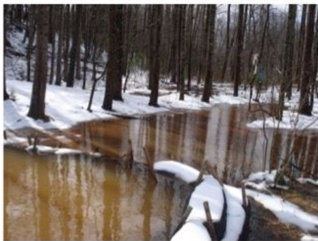
Figure 5: Images showing muddy water overrunning silt socks at the Cahas Mountain Road crossing in late February 2019.
