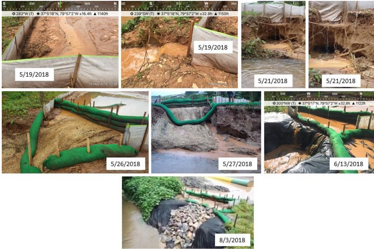
Figure 6: Sequence leading to bank failure on Teels Creek.
